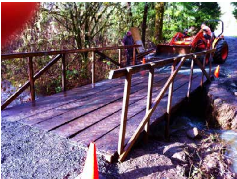
Temporary bridge constructed to provide egress and access to caretakers.
