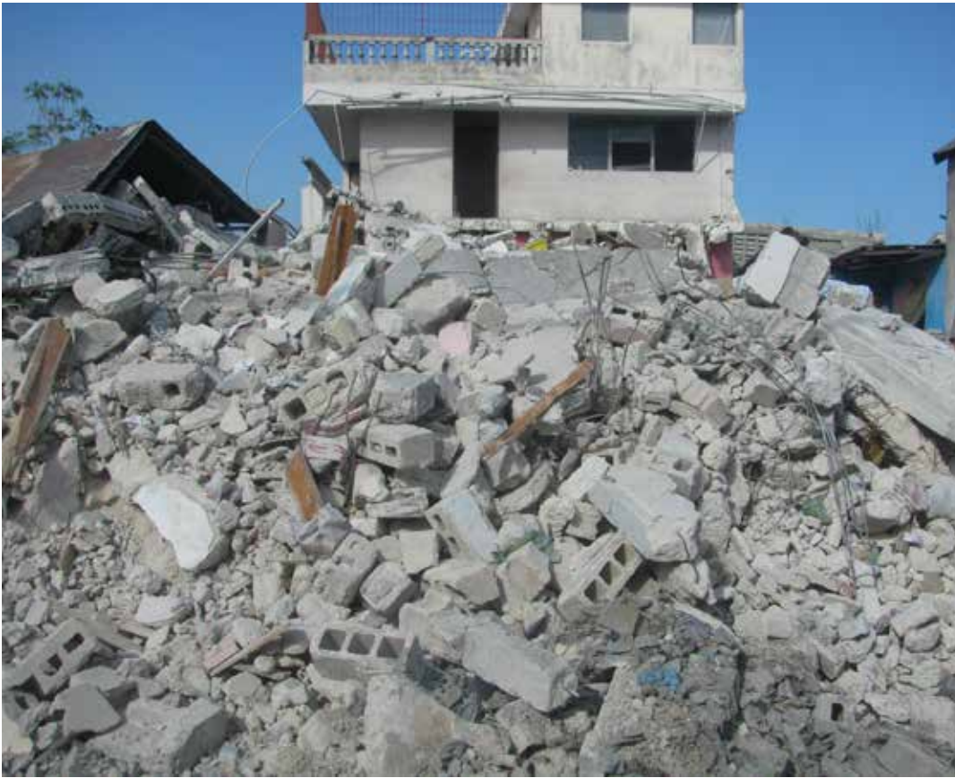
One of many areas devastated by the Haitian earthquake of 2010.
