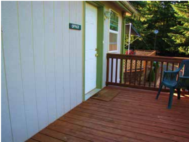
Main office building
