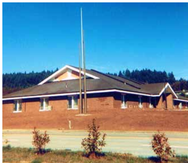
Nearly completed Walnut Building
