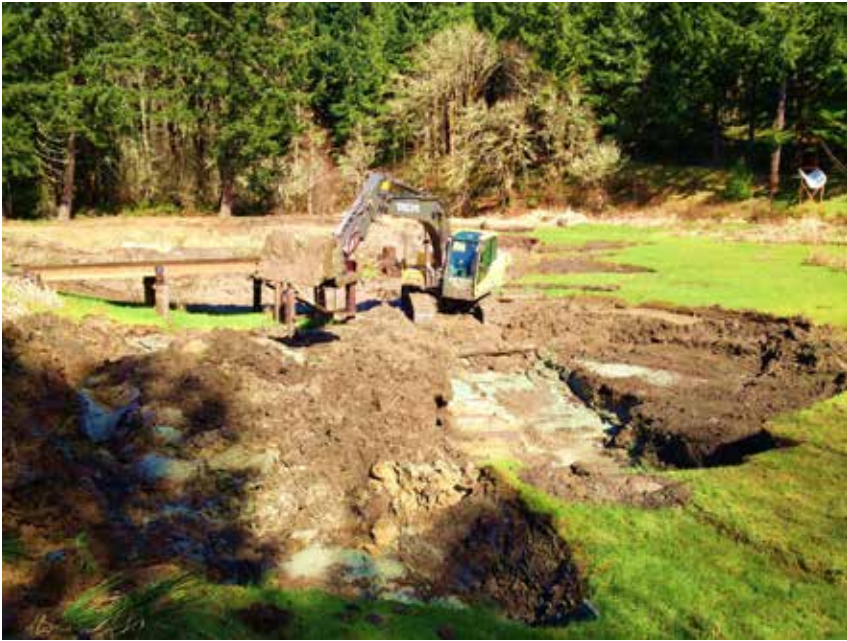
Excavation of mud from the pond.
